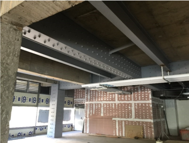
▲ Strengthening the beams with steel plates
