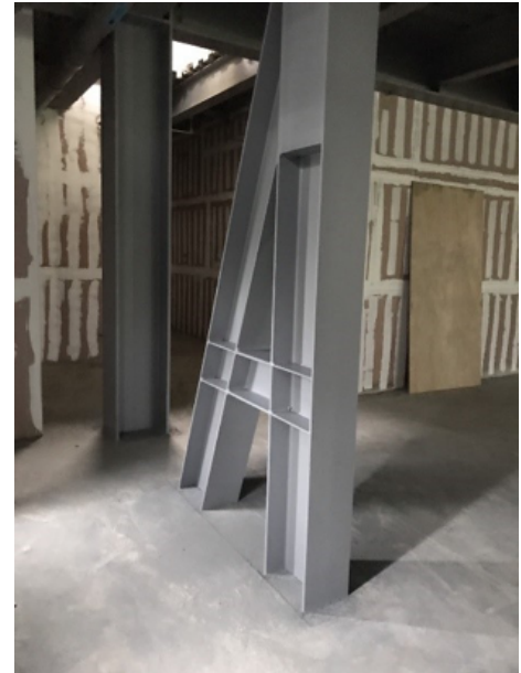
▲ Damper is added
